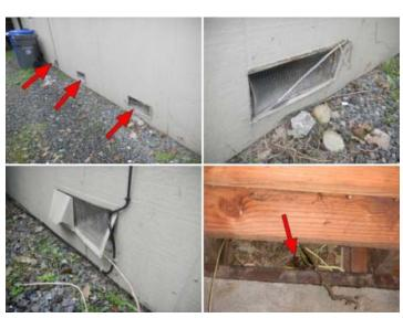
One or more foundation vent screens are damaged or missing. This may allow rodents and animals access to the under-floor crawlspace. Recommend repairing any openings in the screens.
