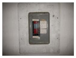
**PROTECTION TYPE:** Overload protection is provided by circuit breakers.
