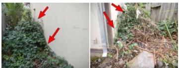
The siding at the left side of the house is observed to be pulled apart at one of the connection seams. I am unable to determine the cause of this condition.
