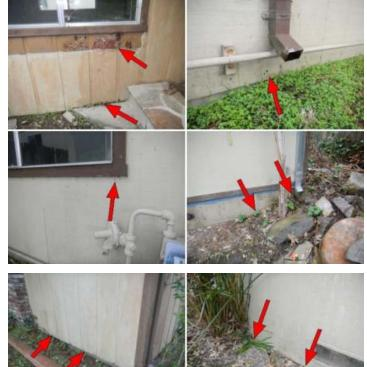
Siding is weathered in some areas around the structure. Wood members were noted which are in contact with the soil or concrete. This condition will have an adverse affect on the duration of wood components. It is recommended to have adequate separation between the ground and siding components.
