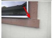
Wood members were noted which are in contact with the soil or concrete. This condition will have an adverse affect on the duration of wood components. It is recommended to
