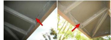
One or more of the rafter tails are deteriorated from moisture in the same areas as the deteriorated roof sheathing. Recommend having this condition evaluated and corrected by the appropriate qualified trades person.
