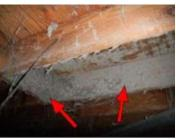
The dryer vent ends or is disconnected in the crawlspace and does not extend to the exterior of the structure. This not only allows excessive moisture to be exhausted under the structure, but the accumulation of lint is a Potential Fire Hazard. Recommend having this condition evaluated and corrected by the appropriate qualified trades person.
