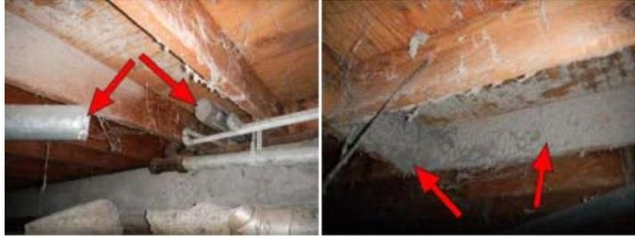
The dryer vent ends or is disconnected in the crawlspace and does not extend to the exterior of the structure. This not only allows excessive moisture to be exhausted under the structure, but the accumulation of lint is a Potential Fire Hazard. Recommend having this condition evaluated and corrected by the appropriate qualified trades person.
